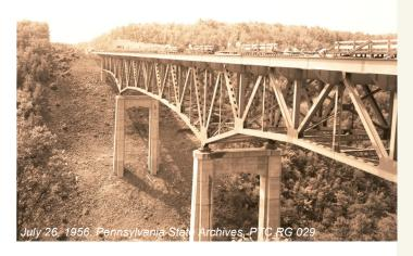
The Hawk Falls Bridge is 738-feet long and the superstructure was made up of five spans: three continuous haunched Warren deck trusses with span lengths of 168, 280 and 168 feet and two secondary simple stringer spans of 68 and 49 feet.
