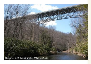
The existing bridge is scheduled for replacement because it is nearing the end of its design service life and considered functionally obsolete due to lack of roadway shoulders.
