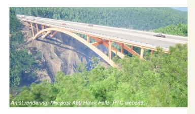
The replacement Hawk Falls Bridge will be a 720'-long steel structure featuring a 480' deck arch span flanked by four 60' deck plate girder spans.
