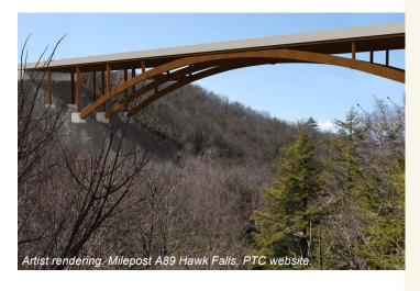
Three welded, steel box arch ribs will be utilized that spans the deep Mud Run Valley located within Hickory Run State Park.
